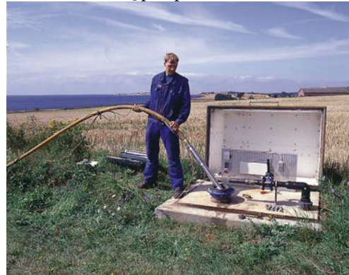
Figure 11. The SQ pump under installation
